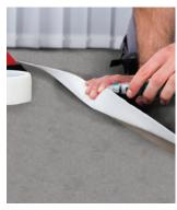
It is important to ensure that all seams between the lengths of underlay butt together. Where an overlap is present this will sit neatly under the adjoining edge.
