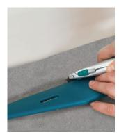
Roll out the selected underlay and trim any excess so that the ends and sides fit neatly against all walls.
