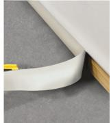
Ensure that the permimeter of the installation is sealed with waterproof tape, running the tape at least 20mm up the walls.
